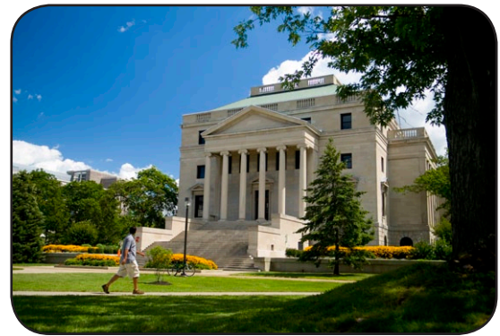
Abbott Hall, South Campus
